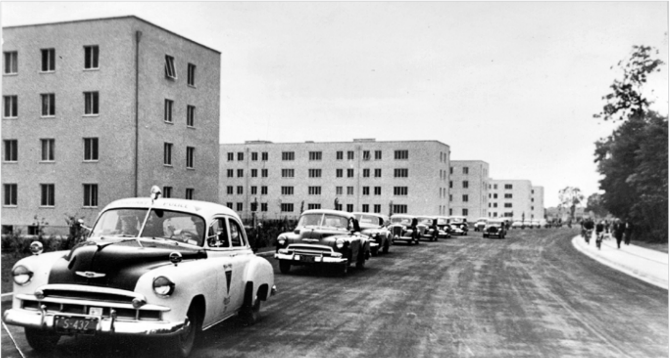
Vorfeld housing along the Ringstraße (StANU, Mangold Collection)
